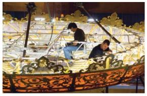
spots or shadows from the fixture's trusswork. This approach eliminated the need for optics by relying on module placement as well as the LUXEON K2's 160-degree radiation pattern for proper light dispersal.
