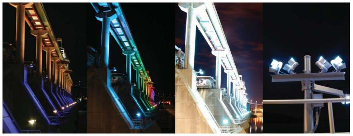
Second, the LUXEON LEDs give the lamps a life expectancy of at least 50,000 hours compared to only 10,000 to 15,000 hours for a metal halide solution. Given the number of fixtures and the challenges of changing them in the Big Dam Bridge's outdoor environment, this dramatically reduces both replacement costs and maintenance requirements.
