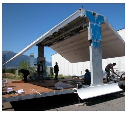
The external surface is covered with stainless steel and sheet aluminium, while the stage itself is surfaced with teak wood decking. The Podium is accessible in front via a broad flight of steps, with separate handicap access. Apart from the mechanisms moving the wings, the cover contains an infra-red heating system and LUXEON-based lighting exclusively planned and produced by Italian manufacturer Space Cannon for the Podium.
